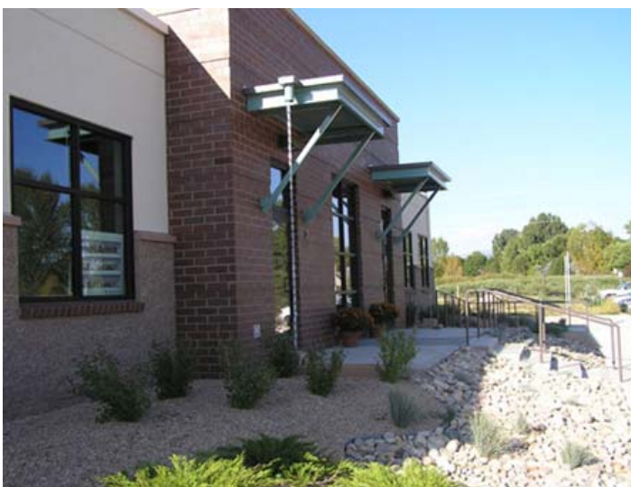
Careful window selection provides daylighting and views while minimizing unwanted heat gain.
